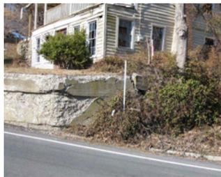
The State's right-of-way will be "shaved" back on the NE corner to improve sight lines down Rte 82 from Rte 7, as simulated in the photo below. The retaining wall between the Tinsmith House and Porter's Store will also be stabilized.
